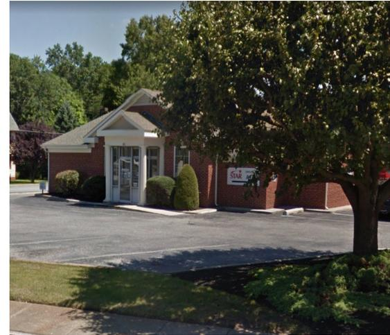
Parking spaces east and west of the bank can be replaced with pervious pavement to capture and infiltrate stormwater runoff from the remainder of the parking lot and rooftop runoff from the bank. A preliminary soil assessment suggests that more soil testing would be required before determining the soil's suitability for green infrastructure.
