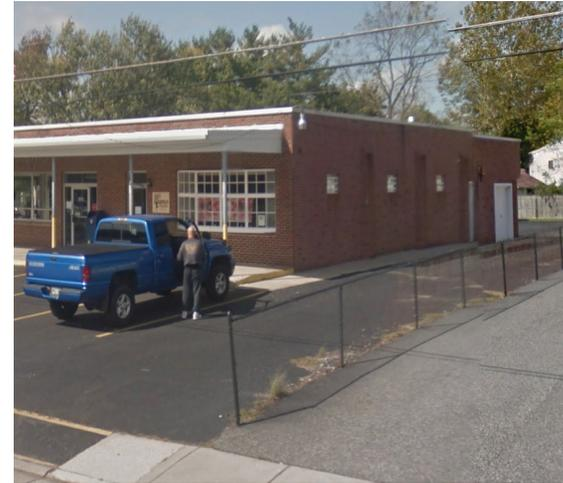
Parking spaces southwest and southeast of the post office can be replaced with pervious pavement to capture and infiltrate stormwater from the parking lot and rooftop runoff from the building. A preliminary soil assessment suggests that the soils have suitable drainage characteristics for green infrastructure.
