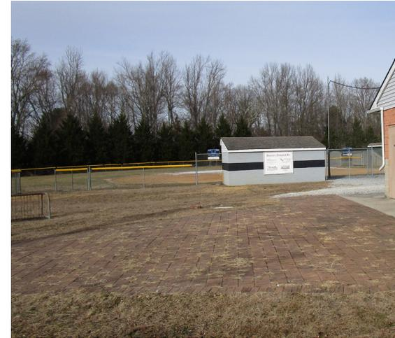
Parking spaces in the middle and northeastern parts of the lot can be replaced with pervious pavement to capture and infiltrate stormwater runoff from the remainder of the lot and rooftop runoff from the nearby building. A preliminary soil assessment suggests that the soils have suitable drainage characteristics for green infrastructure.
